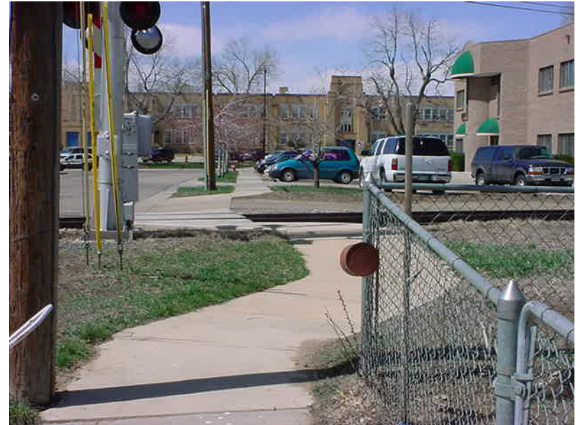
At grade pedestrian railway crossing on Griffith Street
