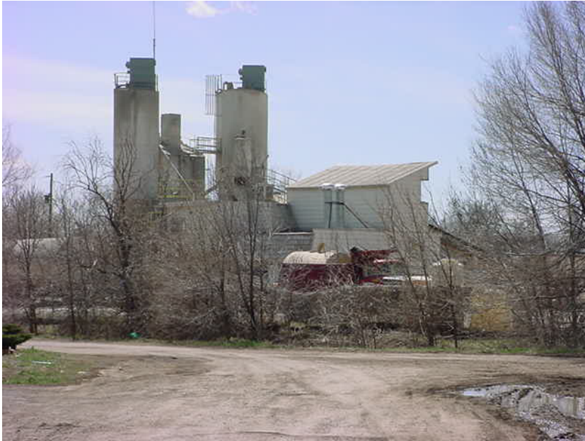
A concrete batch plant occupies a major portion of the Highway 42 Revitalization Area Core
