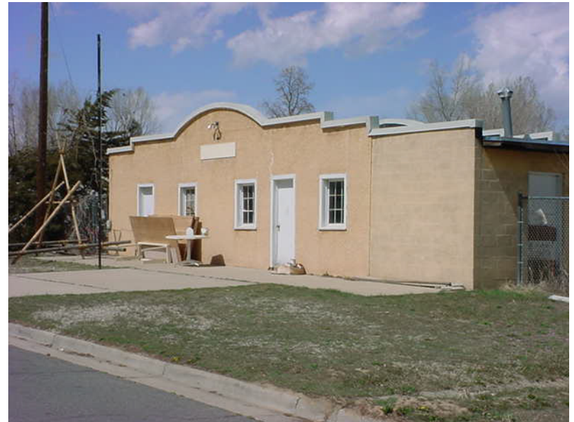
Structure historically used by the Louisville Rod and Gun Club along South Street eligible for historic designation
