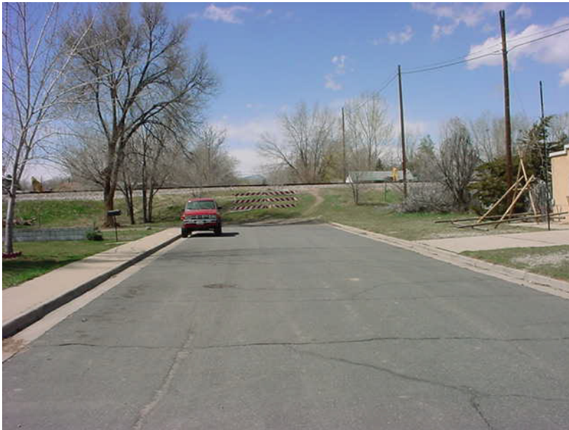
South Street looking west towards Historic Downtown Louisville
