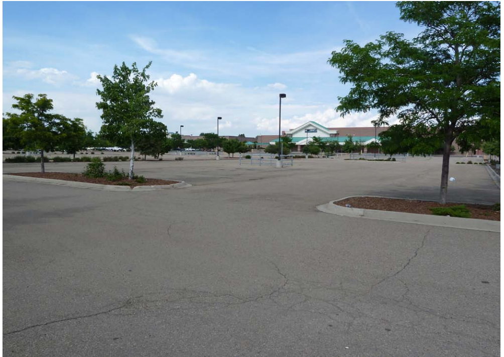
The vast parking area and the building lie largely vacant
