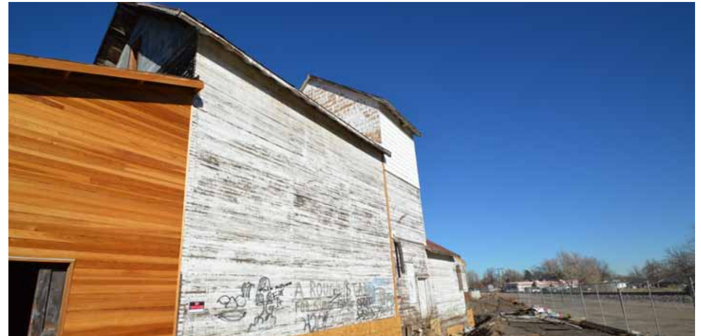
Louisville Grain Elevator
