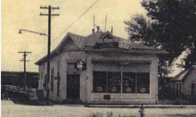
The Di Francia Saloon was built in 1904 at the corner of Front and Spruce Streets. Operating under several different names over the years, this photo from the 1948 Boulder County Assessor’s card shows it as the Colorado Café.
