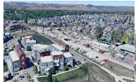
VIEW FROM THE SOUTHEAST
