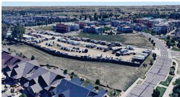
VIEW FROM THE NORTHWEST
