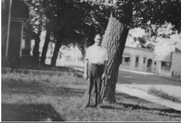
This Moffitt photo is believed to show, on the left, the rear of the south part of 641 Main.
