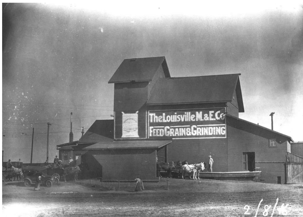
Louisville Grain Elevator, 2/8/1916, Louisville Historical Museum
