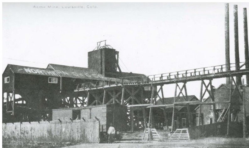
The following photo has a view looking east and shows the engine house, boiler house behind it with three smokestacks, fan house, and the Louisville Grain Elevator in the distance.
