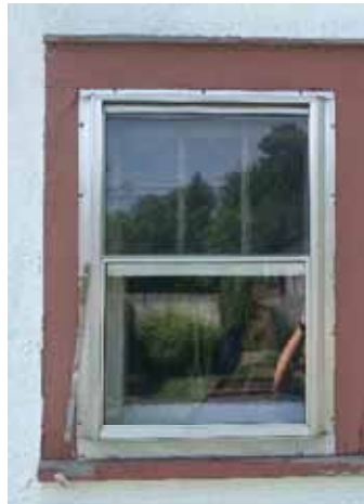
Original window and aluminum storm window
