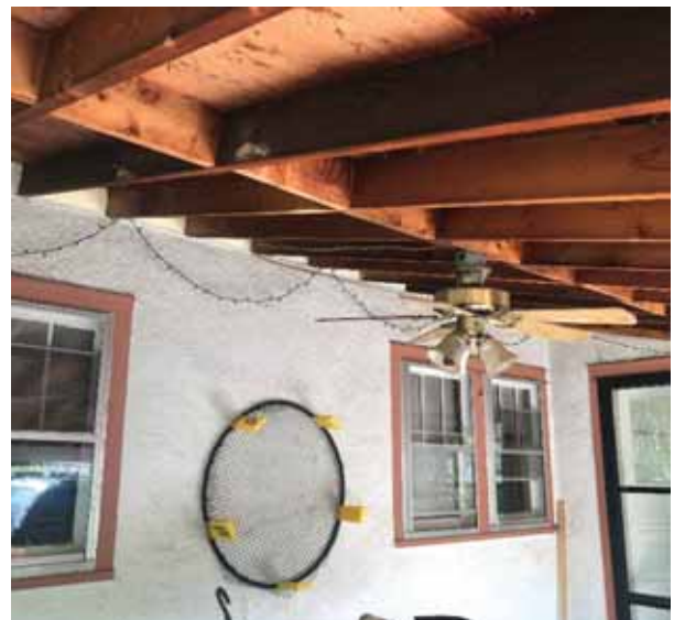
Shed roof framing over patio in southeast corner of the house.
