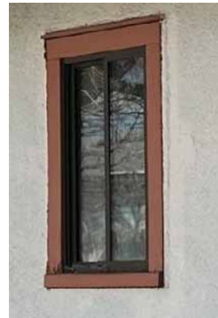
Replacement aluminum slider window.
