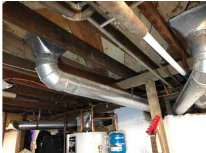
Floor joist supports were added where the foundation wall was opened up.
