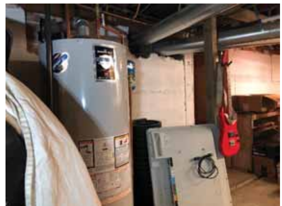
Central foundation wall with openings for ductwork.
