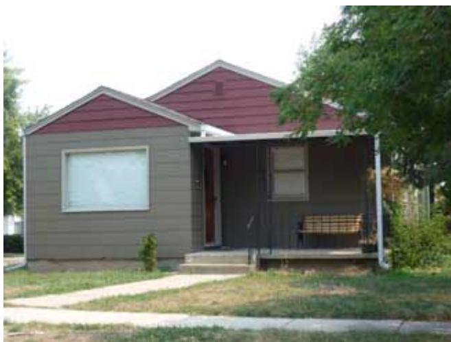
Current Boulder County Assessor photo of 1440 Cannon.
