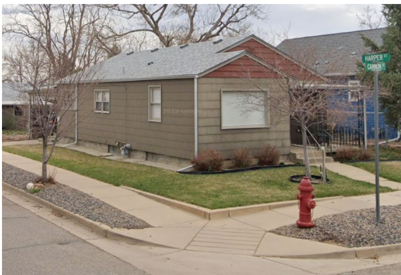
Figure 2. Recent streetview from Cannon and Harper intersection.
