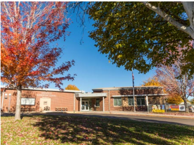
3 Louisville Elementary School (Source: Boulder Valley School District)
