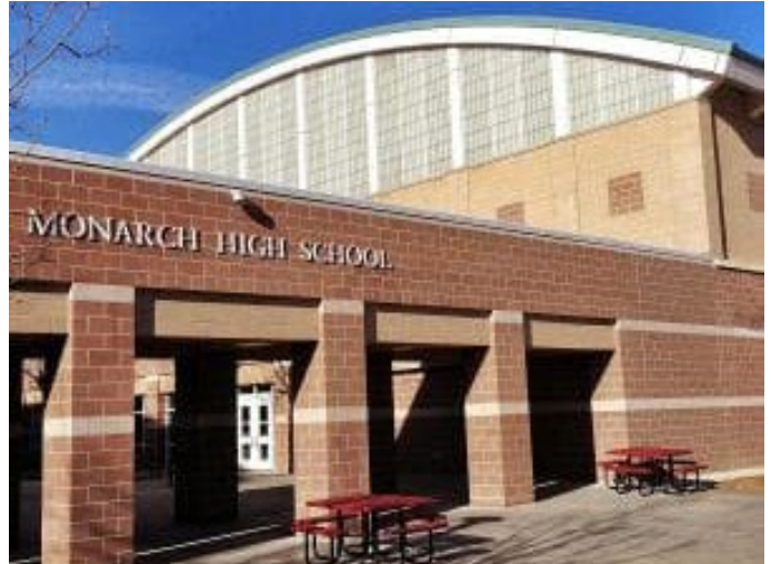
4 Monarch High School (Source: Boulder Valley School District)
