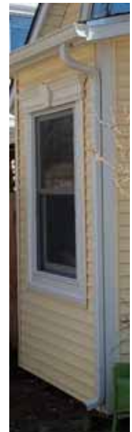
Typical gutter & downspout without an extension
