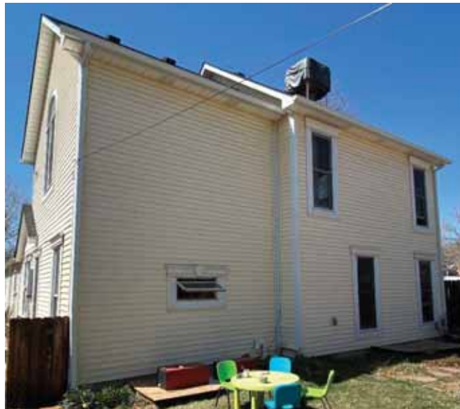
Swamp cooler at back of house
