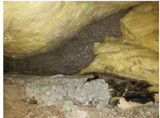
Crawlspace foundation with insulation pulled back
