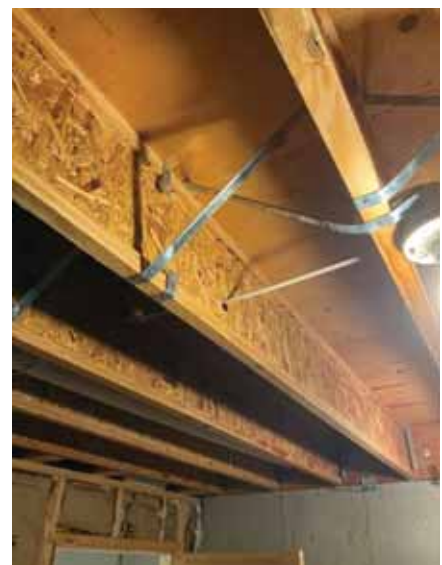
Floor framing in 1995 addition
