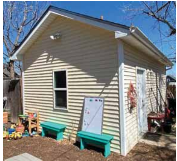
1-car garage as viewed from the back yard
