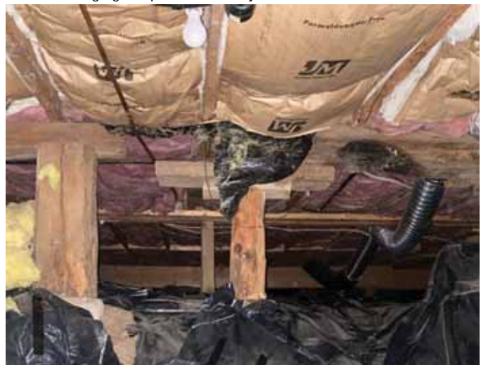
Floor framing and assortment of supports in crawlspace
