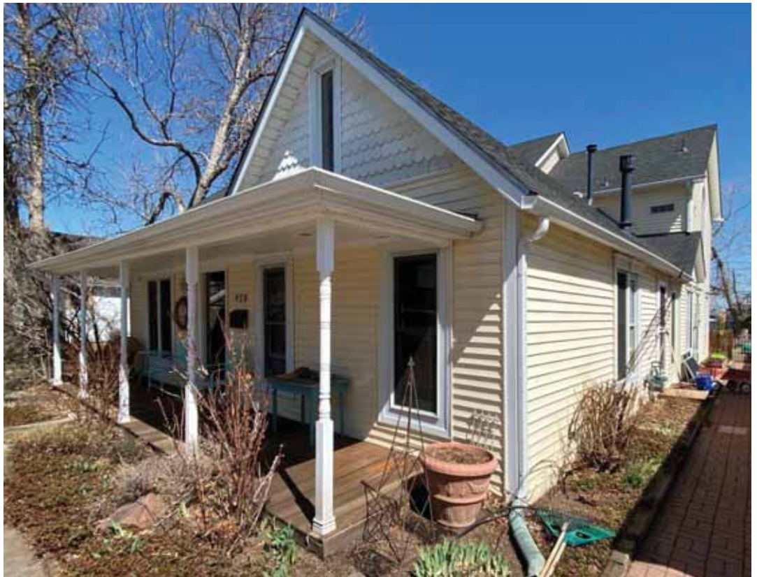
2021 View from the Southwest
