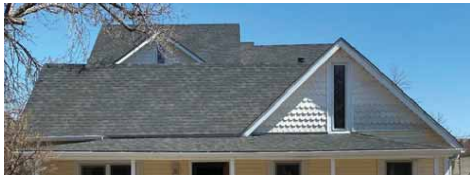
Asphalt composite shingle roof added in 2018
