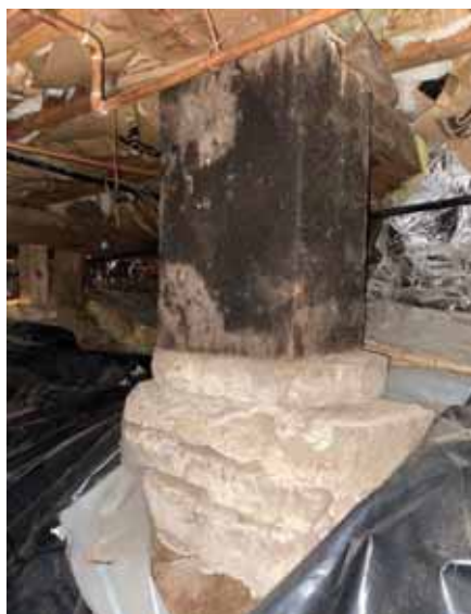
Support column in crawlspace
