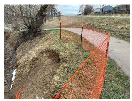
3. At the Kennedy Ave access to Coyote Run Open Space, damage to the area next to the sidewalk was identified. This was caused by recent snow removal efforts. Public works was informed of the matter and plans to restore the area in question with the guidance of the Open Space department. The photos below are provided to show the condition of the area.
