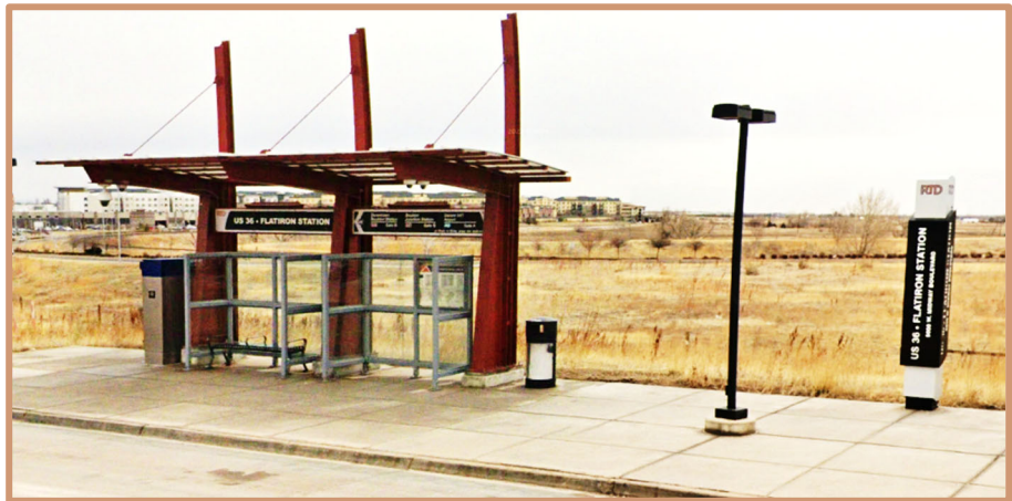
Photo 1: US 36 and East Flatiron Station
