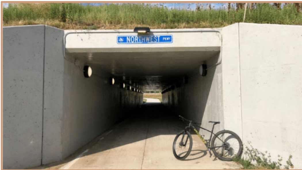
Photo 3: Northwest Parkway Multi-Use Path Underpass
