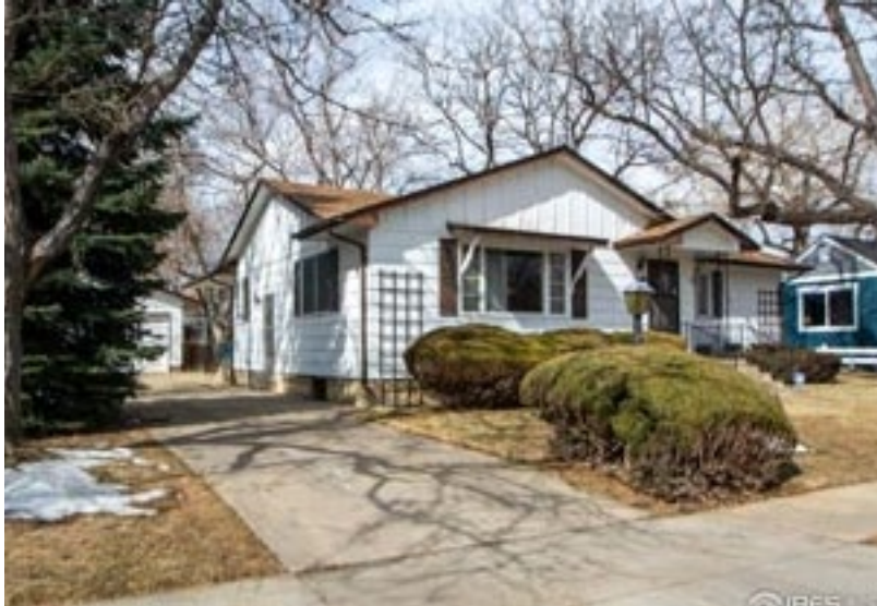
Current Boulder County Assessor photo of 623 McKinley
