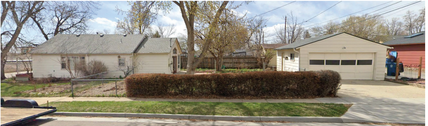
View from Short Street. Side elevation of primary structure at left. Existing garage at right.
