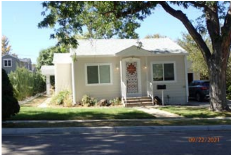
Current Boulder County Assessor photo of 1213 Jefferson.
