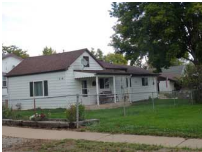
Current Assessor's photo of 516 Grant.
