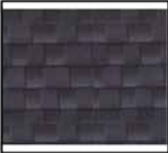
ASPHALT SHINGLE ROOF
