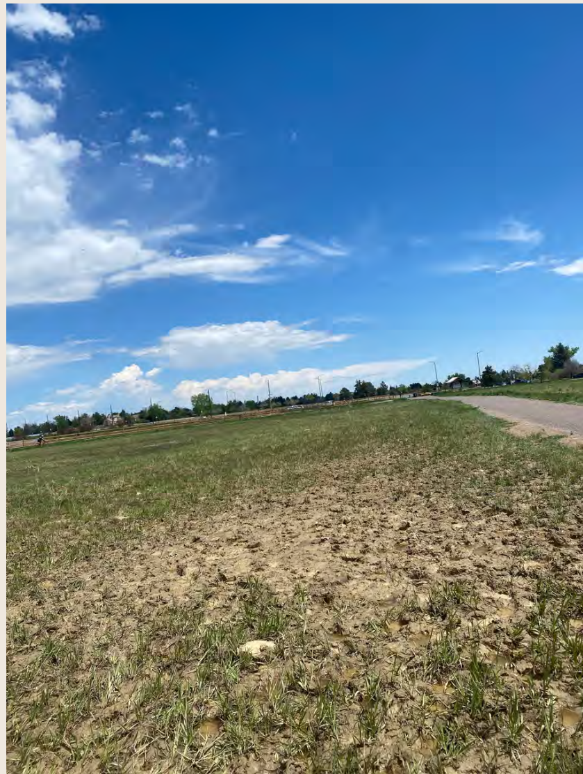
Pugging in Area 1
