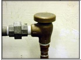
Used mainly on lawn irrigation systems. It has an air inlet valve that will drop to draw in air thus preventing sprinkler system water from entering the City's water mains.
