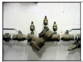
Operates similar to a Pressure Vacuum Breaker. Used on low hazard applications and on fire lines.
