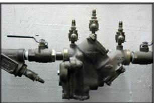
Used on high hazard applications. It is a combination of check valves and an air inlet allowing water from the private system to vent when City pressure drops.
