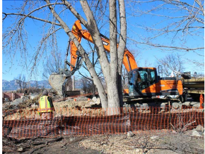
PRIVATE DEBRIS REMOVAL
