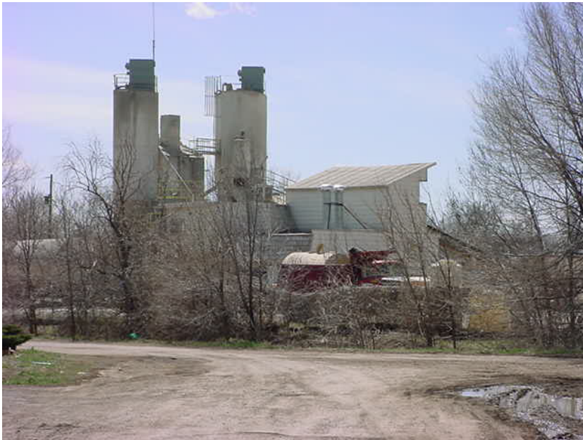
A concrete batch plant occupies a major portion of the Highway 42 Revitalization Area Core
