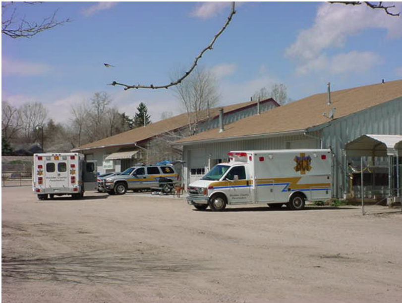
Boulder County Paramedics Facility at Highway 42 and South Street
