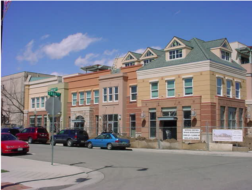
New construction along Front Street in downtown Louisville. The massing and scale is indicative of downtown Louisville buildings. Similar building massing and scale is expected in the Highway 42 Revitalization Area Core.
