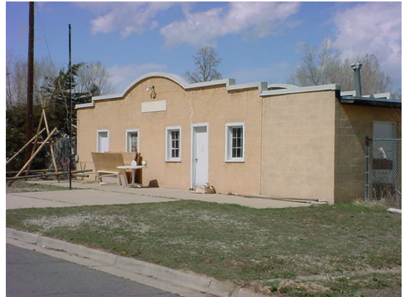
Structure historically used by the Louisville Rod and Gun Club along South Street eligible for historic designation
