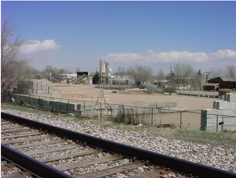
A view of the site intended for an RTD commuter rail platform and park-n-Ride
