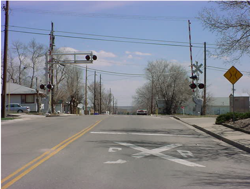
At grade street crossing at Griffith Street
