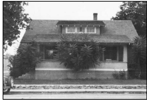
Eberharter House (now the Louisville Chamber of Commerce) at 901 Main St. in 1948. This is an example of a Craftsman style bungalow.
