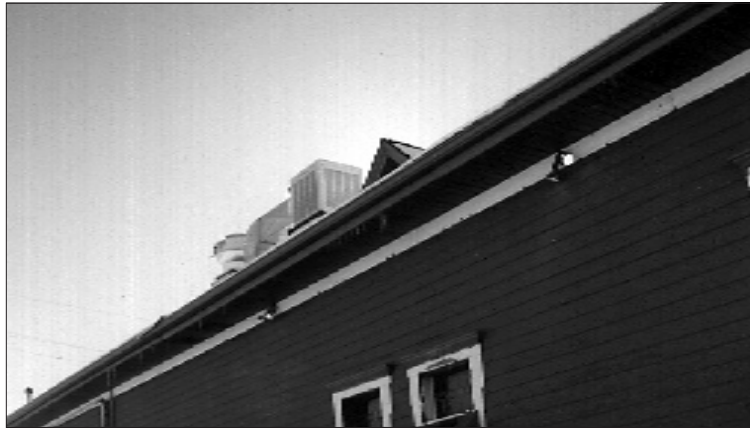
X Minimize the visual impacts of utilities and service equipment
