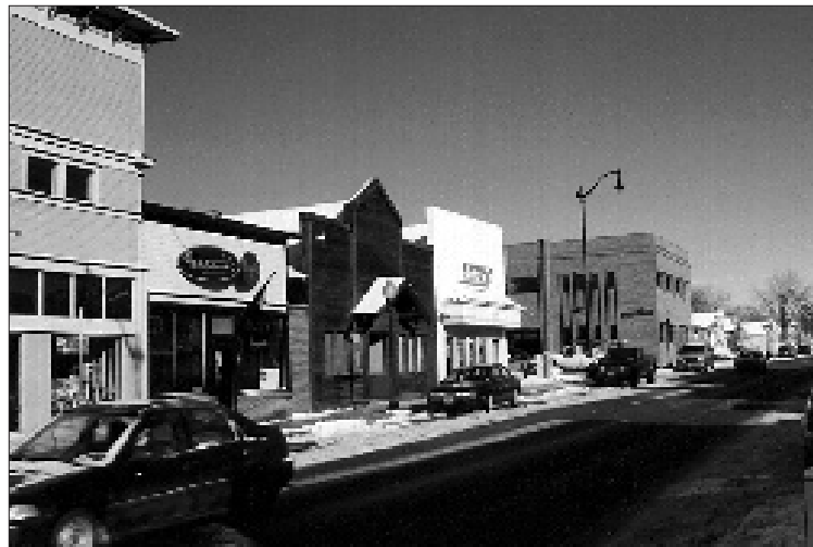
More recent alterations, like these western and southwestern "cover-ups," that are not historically significant may be removed.
