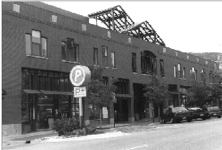
Design a parking structure to allow space for active uses at the sidewalk edge, such as the Spruce Street garage does in Boulder, CO.
