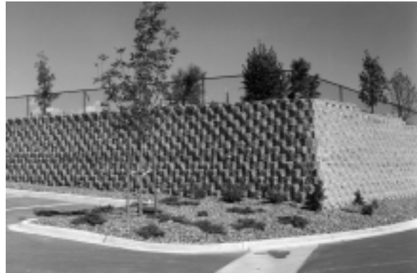
6.1.A - AVOID RETAINING WALLS IN EXCESS OF 30"
