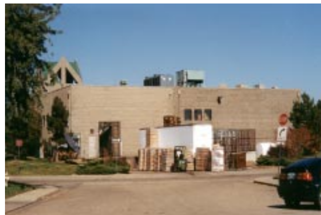
1.6.H - THIS IS NOT PERMITTED - OUTSIDE STORAGE MUST BE FULLY SCREENED
