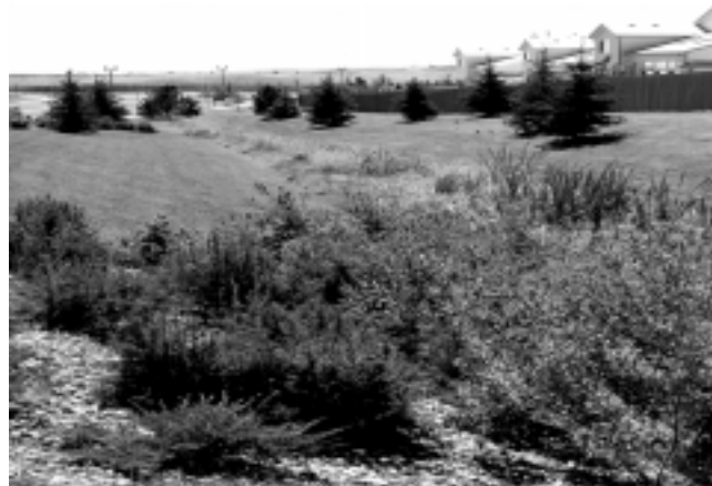
1.7.A - GOOD EXAMPLE OF NATURAL GRASSY SWALE
