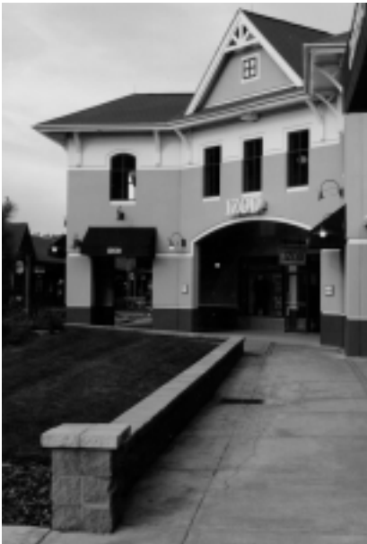
9.9 A INCORPORATE CLEARLY DEFINED, HIGHLY VISIBLE CUSTOMER ENTRANCES FOR EACH PRINCIPAL BUILDING.
