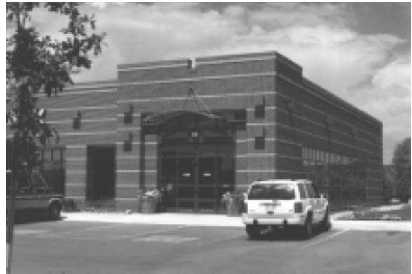
4.3 G USE BUILDING MATERIAL THAT CAN VISUALLY BE MEASURED TO GAIN A SENSE OF HUMAN SCALE.
