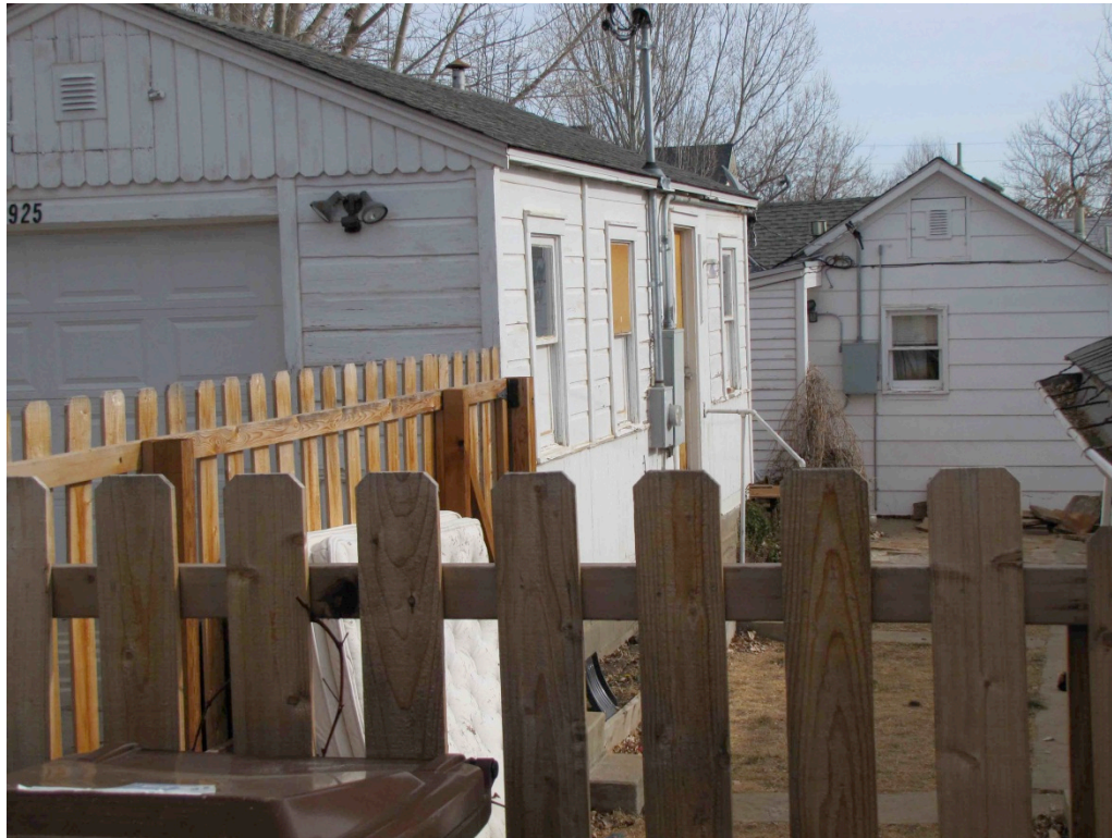
5BL8000_925LaFarge_07 garage south
