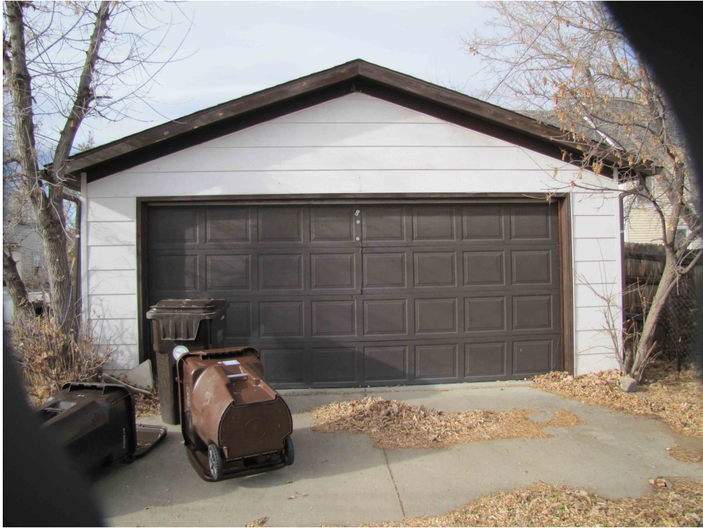
5BL7999_920LaFarge_05 garage east
