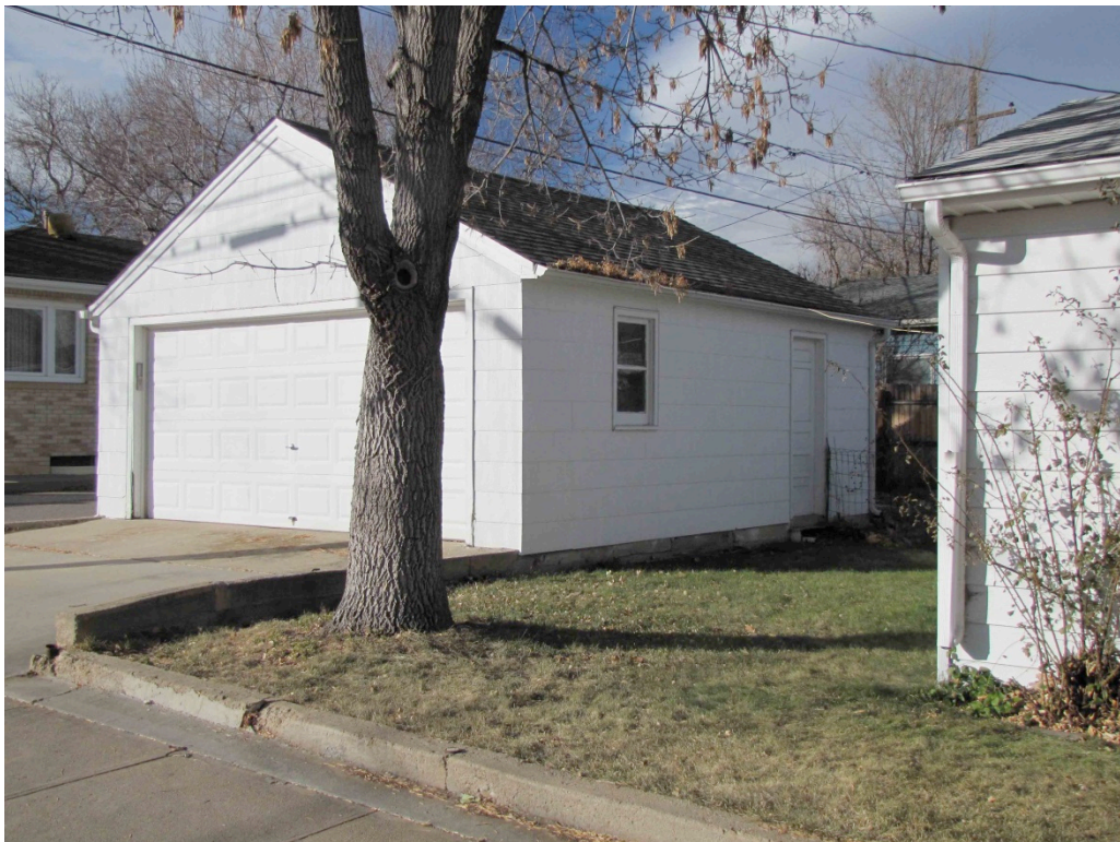
5BL7995_717Walnut_04 garage southeast
