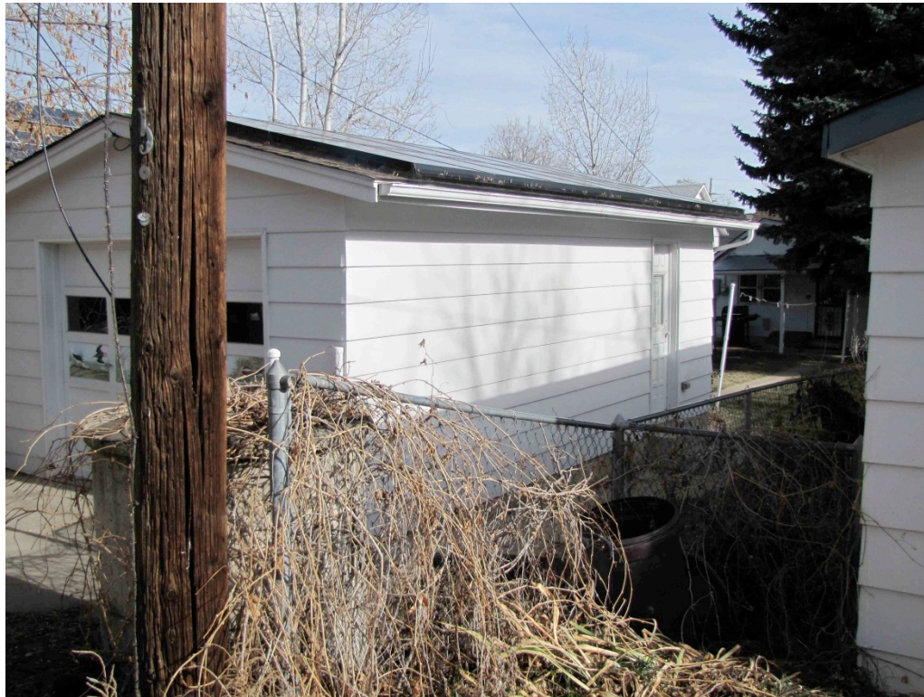
5BL7990_821LaFarge_05 garage southwest
