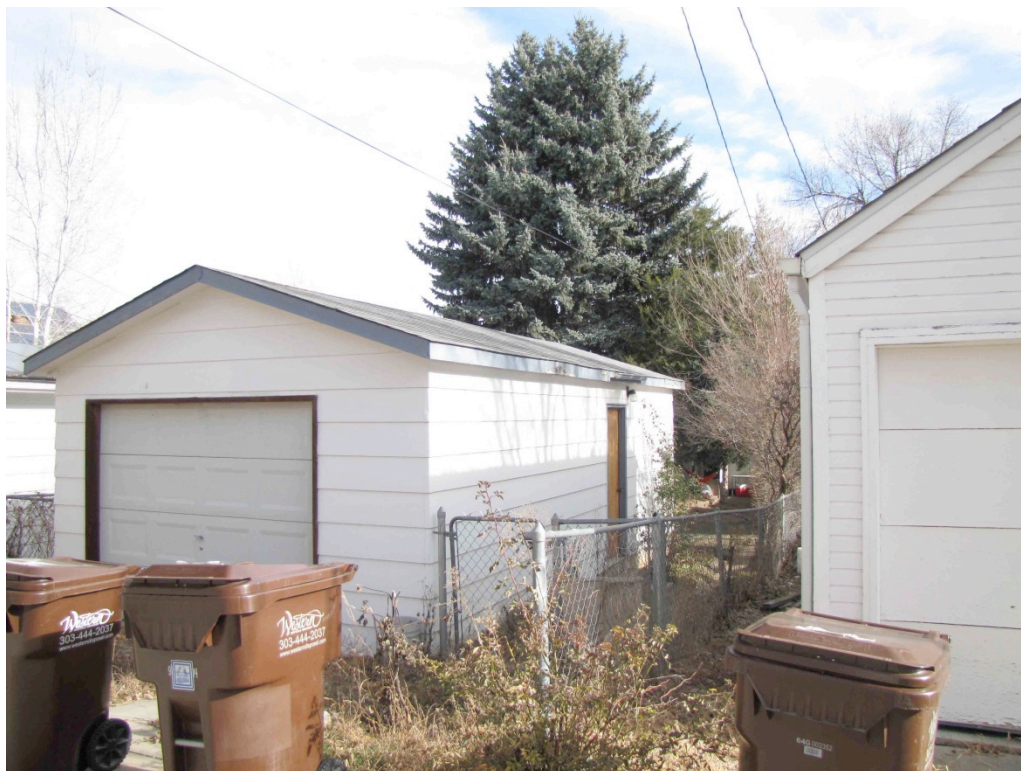
5BL7989_817LaFarge_04 garage southwest
