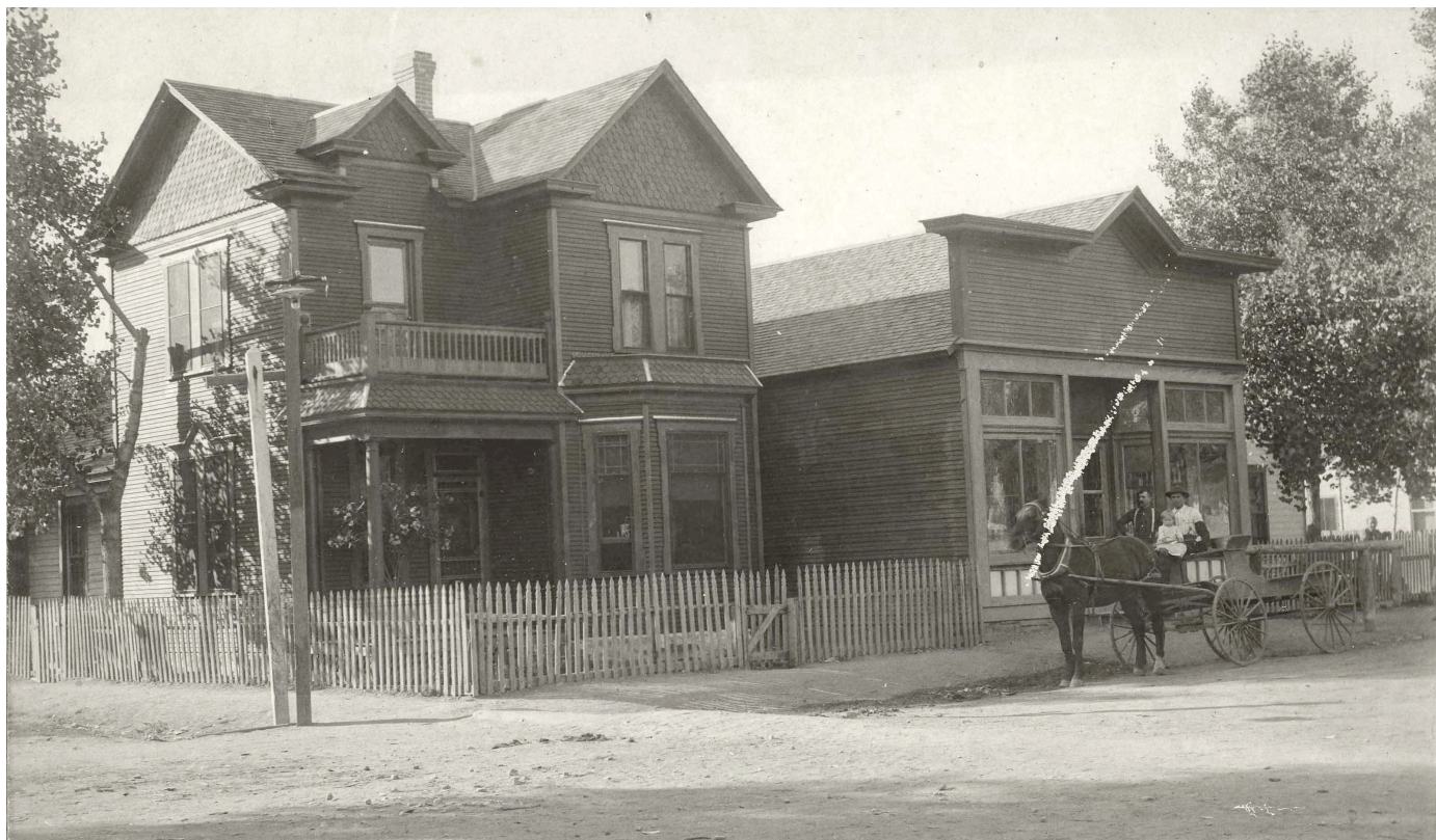
Undated photo, prior to 1931, Louisville Historical Museum 2009.049.004, donated by granddaughter of Martha and Ludwig Eberharter. 801 LaFarge (5BL852) is on the left and 805 LaFarge is on the right.
