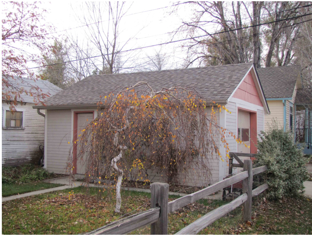
5BL11284_745LaFarge_05 Garage Northeast
