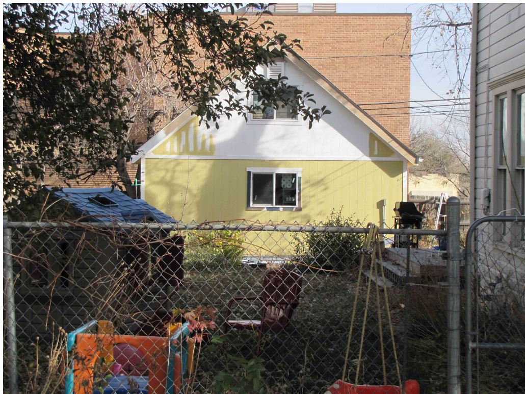
5BL919_728LaFarge_06 Garage East
