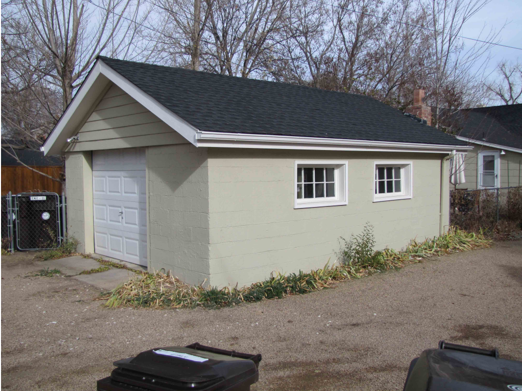
5BL7980_721LaFarge_05 Garage southwest
