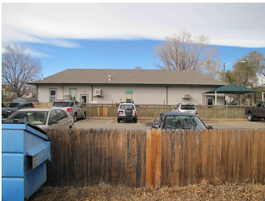
5BL920_628LaFarge_04 East side and parking lot
