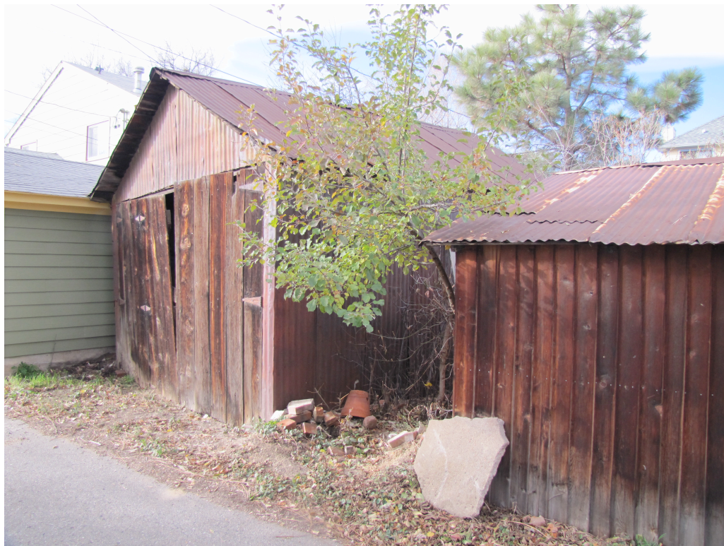
5BL7976_608LaFarge_07 garage northeast
