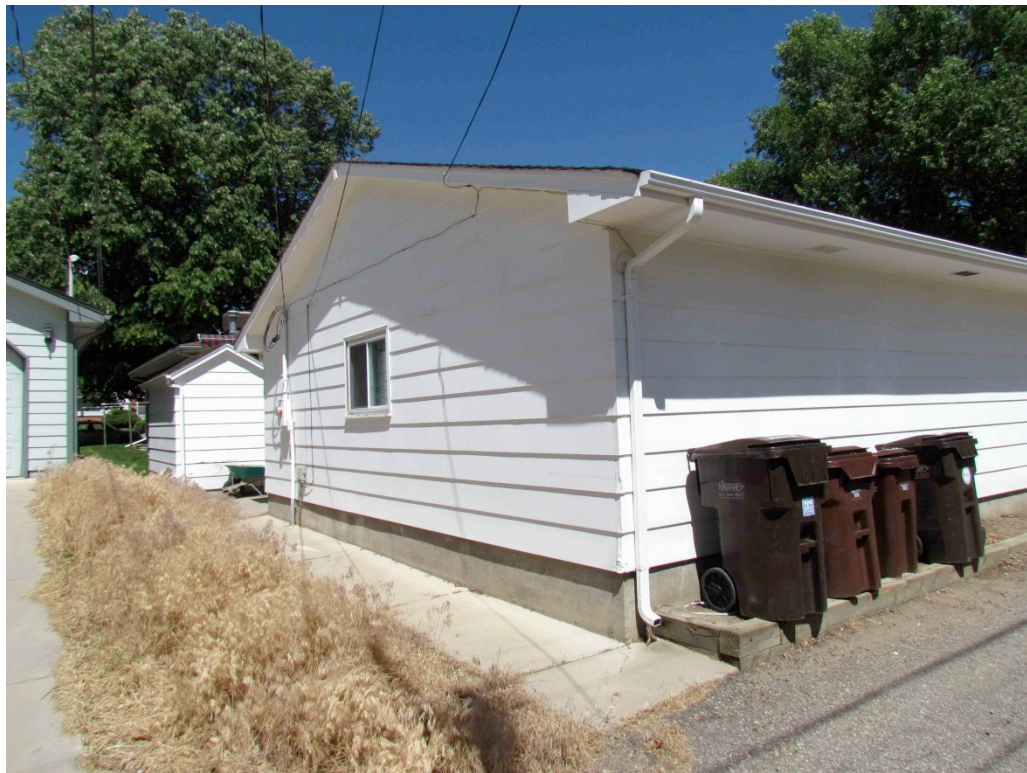
5BL11306_836Jefferson_06 garage south
