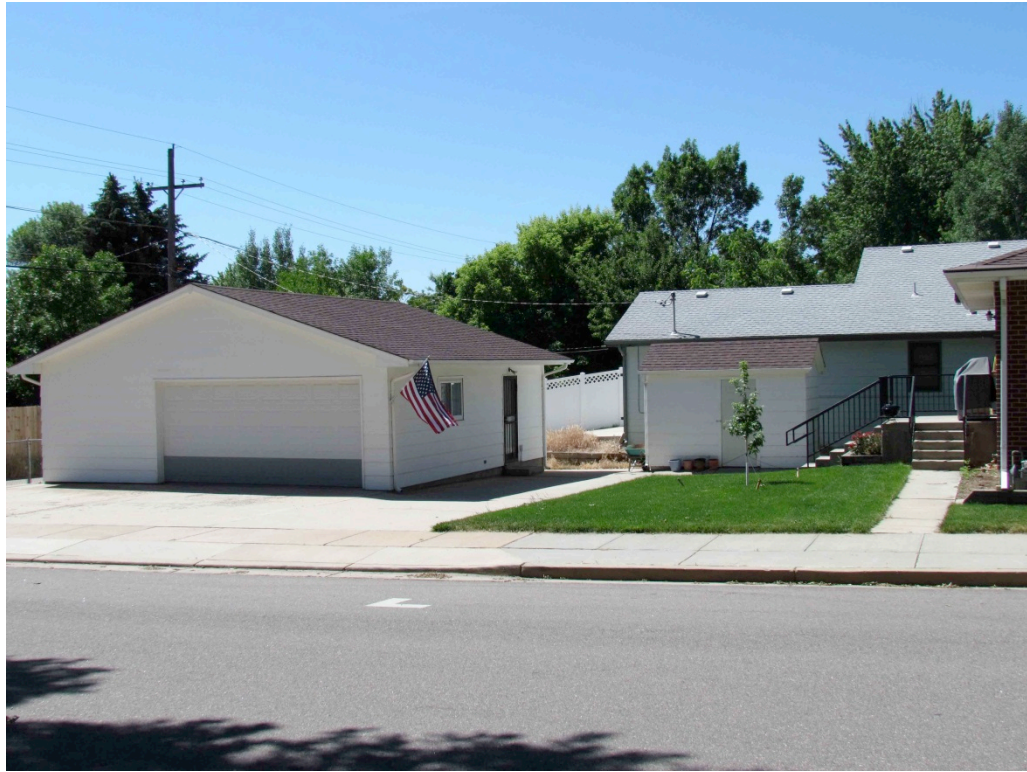
5BL11306_836Jefferson_05 garage northeast
