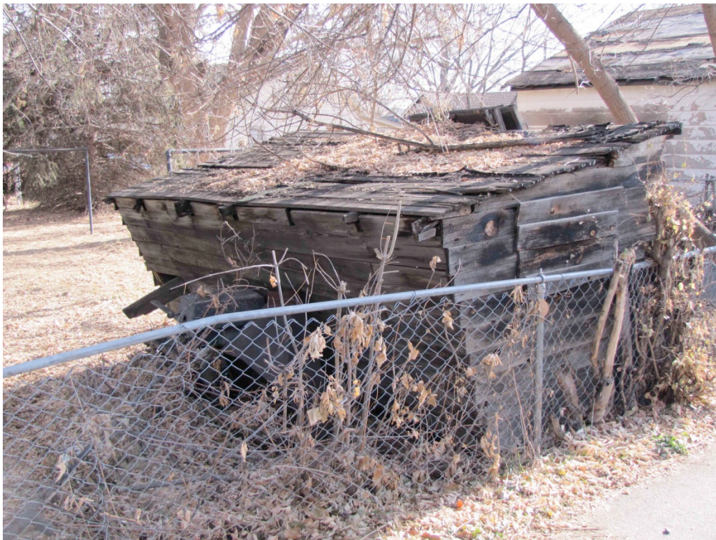
5BL11297_721Jefferson_06 southern shed
