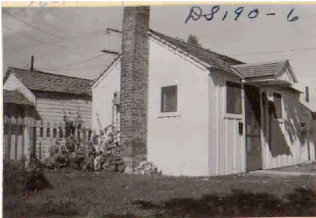
616 Jefferson. Boulder County Real Estate Appraisal card, 1950. Does not resemble the current 616 Jefferson, so the address may have been re-assigned. The pictured building does not appear to still be on this site.
