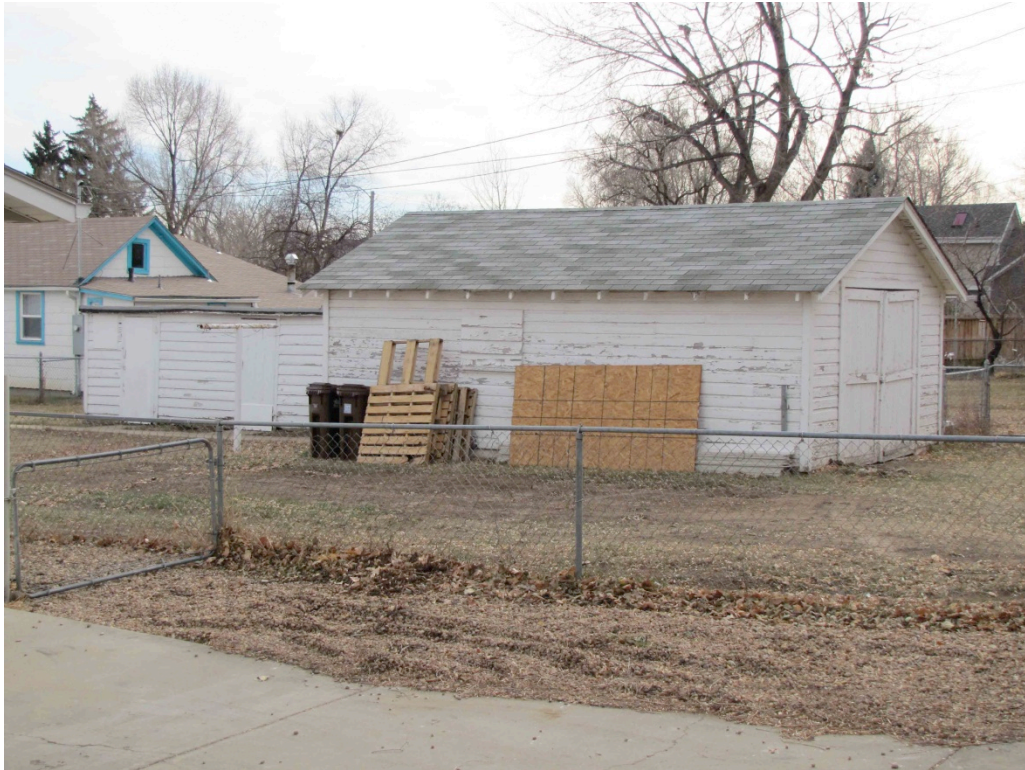
5BL11289_613Jefferson_05 north garage & shed
