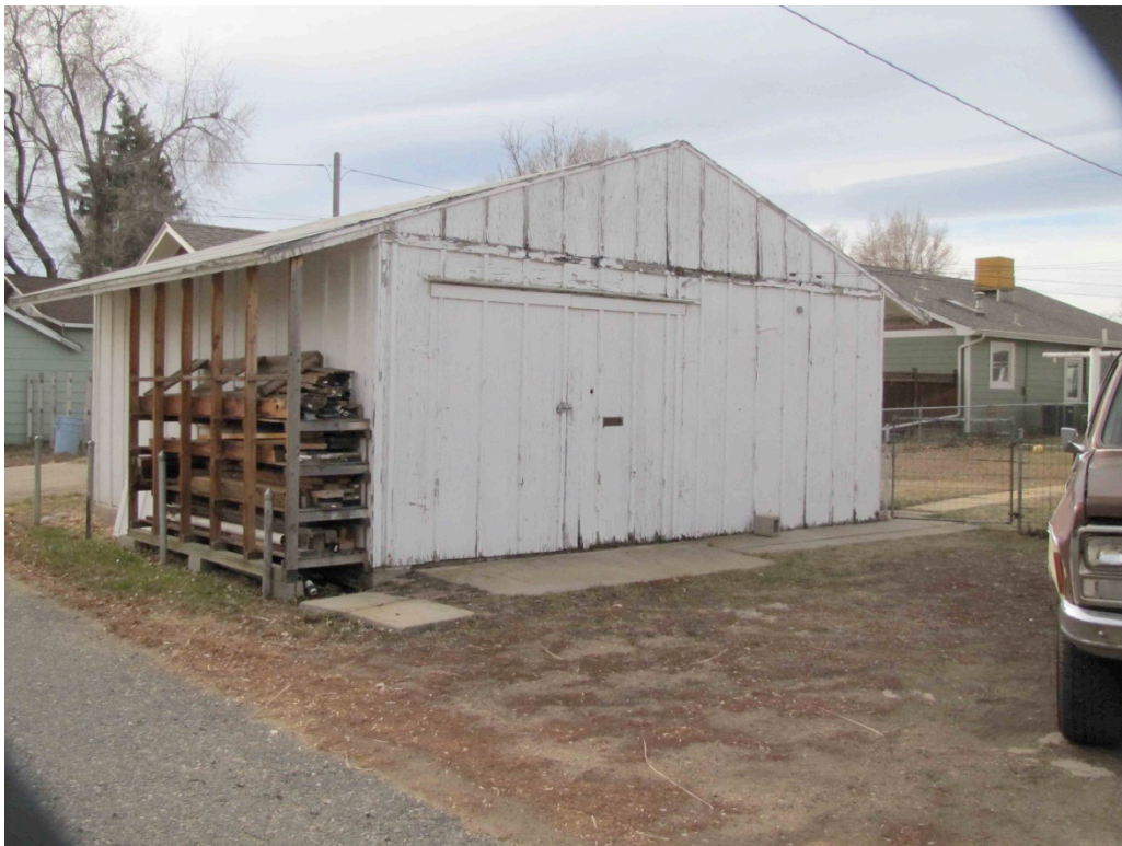
5BL287_600Jefferson_08 barn northeast
