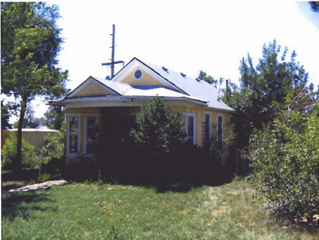
Front and side elevations. Looking southeast.
