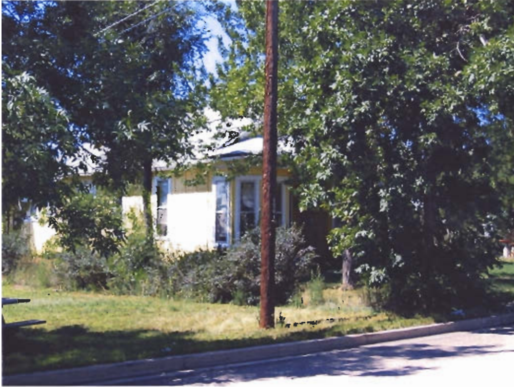
Side elevation. Looking southwest.
