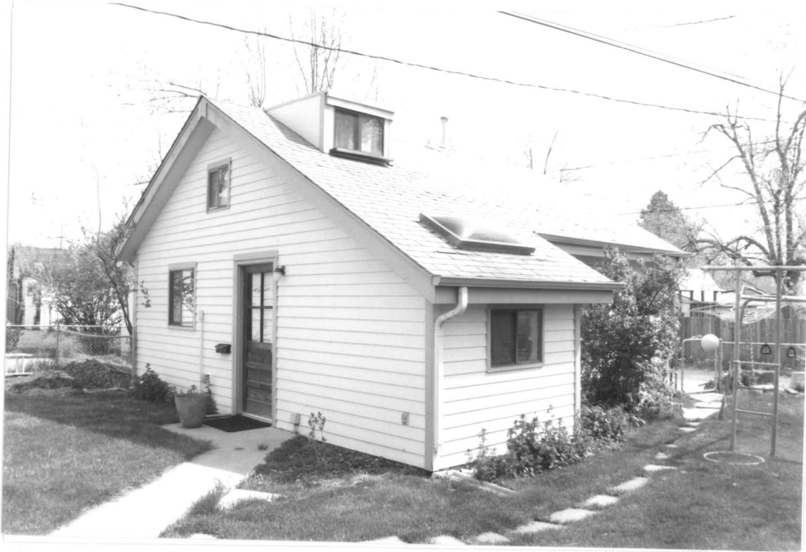
5BL8003 600 Lincoln Avenue, Louisville House 26 April 2000 Negative located at: City of Louisville 749 Main Street, Louisville, CO 80027 Photographed by Carl McWilliams Roll CM-7 Frame 9 View to SE
