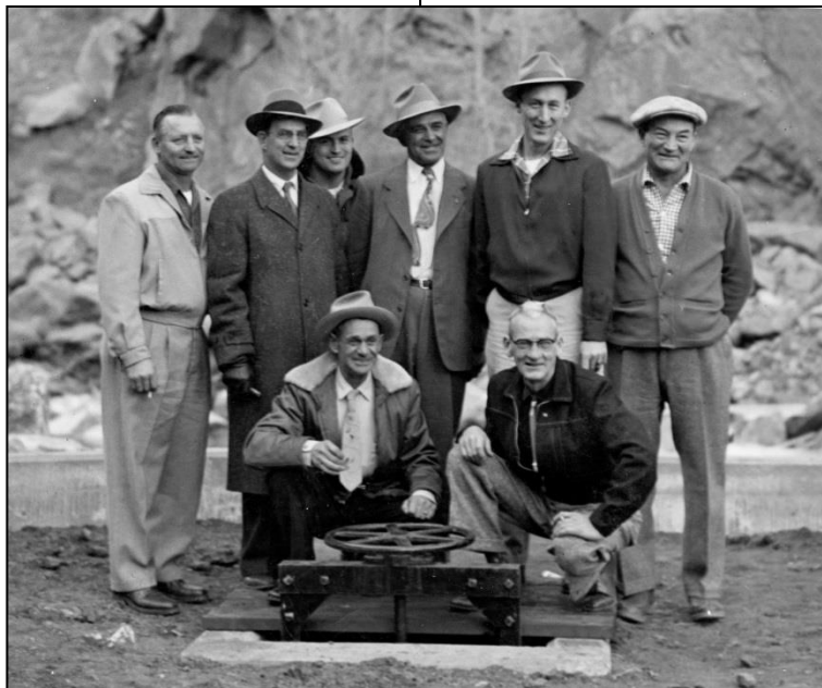
In 1956, a 12-mile pipeline to bring water to Louisville was completed. This photo shows the dedication, believed to be in Eldorado Canyon, with men ready to turn the valve. Kneeling, L to R: Town Clerk Ring Dionigi and Mayor Henry McHugh; standing, L to R: Town Trustee Andy Deborski; Town Attorney Joe Morrato; and Trustees Ray Caranci, Frank Rizzi, Lloyd "Bud" Brown, and Gene Madonna.
