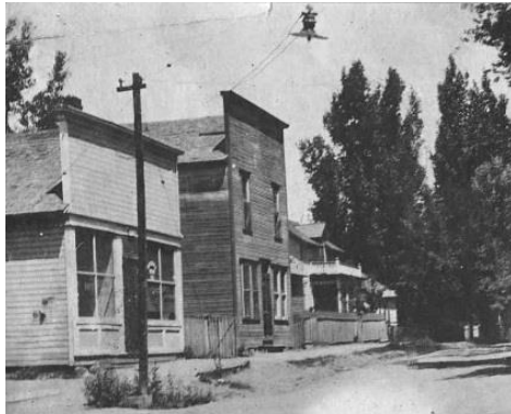
Original two story building next to Jacoe Store, where a Visitor Center is envisioned.
