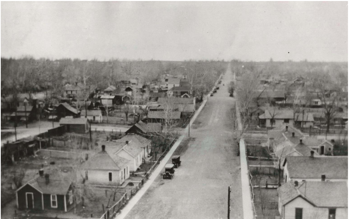
View from Acme Mine dump, looking north on Main Street.
