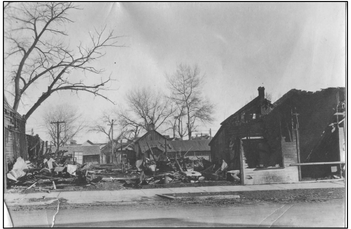
It appears that this photo was taken after the burned debris from the Telephone Exchange building was taken away.
