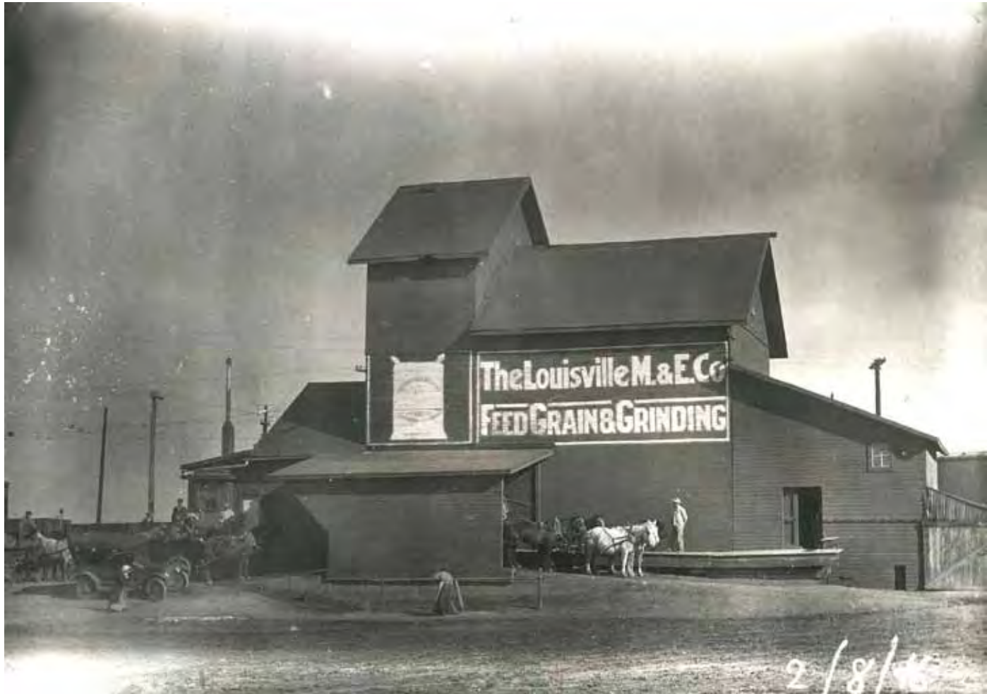
Louisville Grain Elevator, 1916
