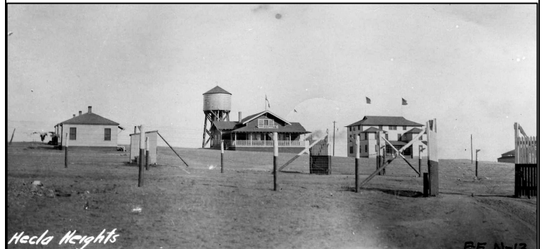
Fenced enclosure with Hecla Mine buildings, circa 1910-1915. From left to right are miners’ housing, water tank, the “Casino,” and the boardinghouse. The Casino building, built for the recreation of strikebreakers and to keep them in the enclosure, is still standing at 1800 Plaza Drive.
