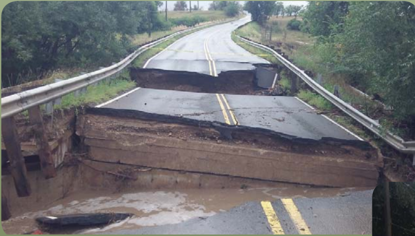
County Road Bridge September 2013
